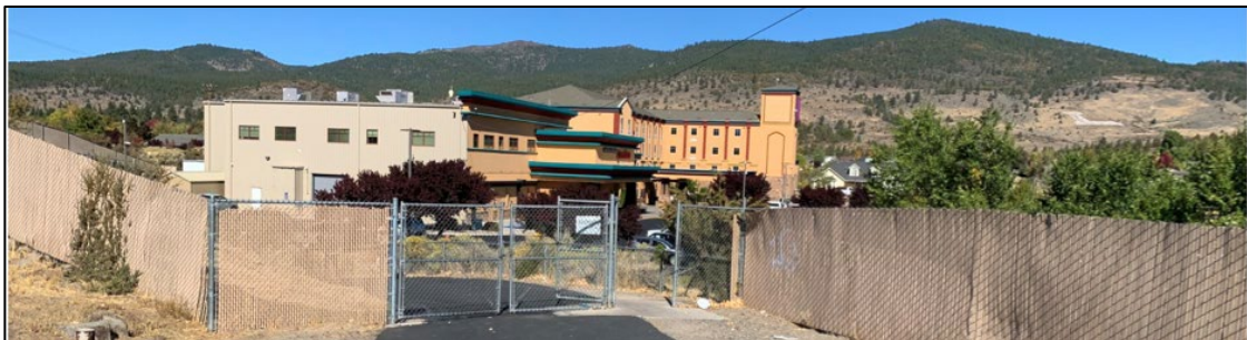
Figure 4-5: End of San Joaquin Street, Pedestrian Access to the Casino
