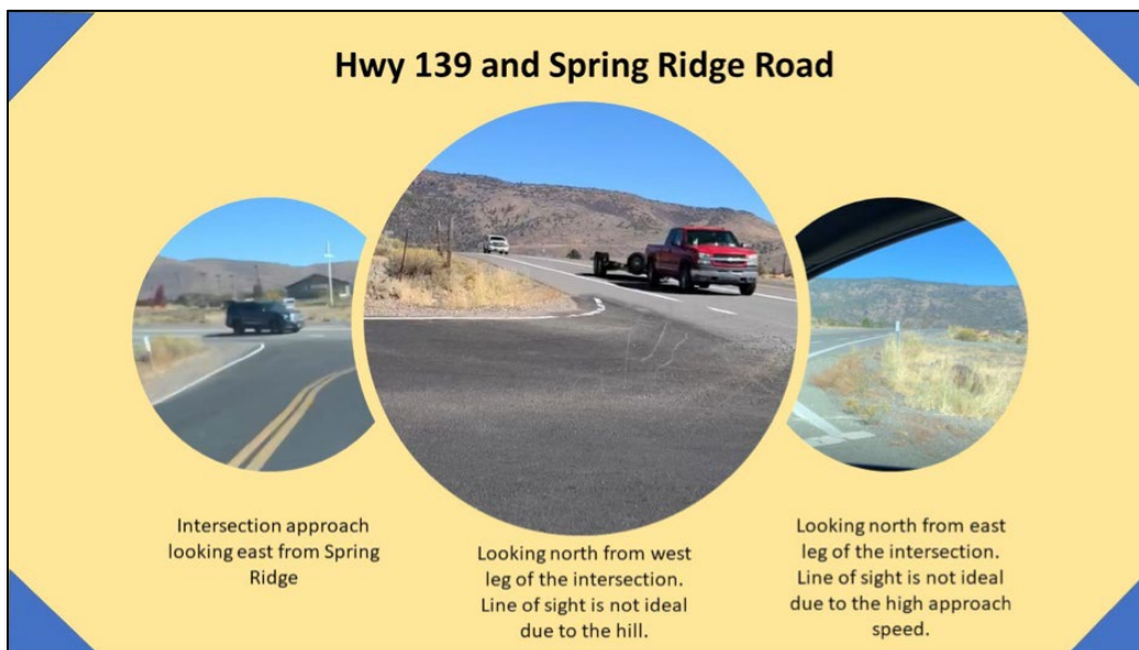
Figure 4-8: Intersection of Hwy 139 and Spring Ridge Road Views
