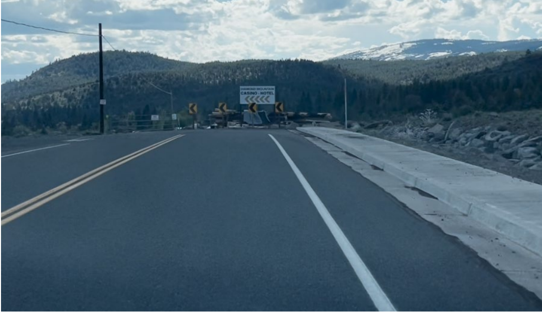
Figure 4-11: Spring Ridge Drive end at Numa Road Intersection
