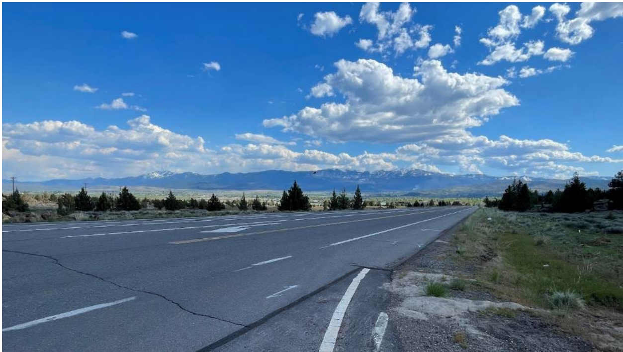
State Highway 139 at Spring Ridge Drive. Looking South.
