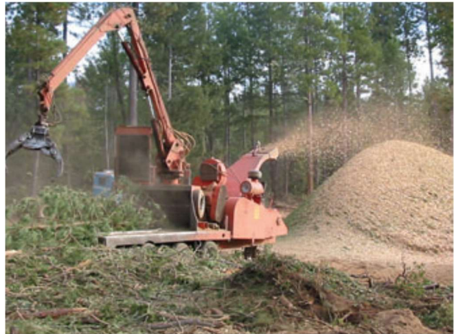
Figure 17. Removal by chipping -One method to remove slash from the site is to use high powered chippers and trucks to haul material to utilization or disposal sites.
